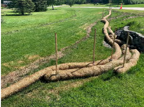
29 Gundalow - 1 (Drainage Area)
