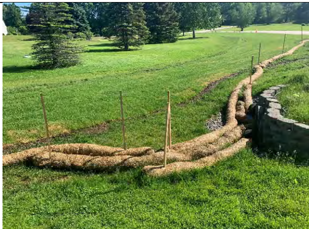
29 Gundalow - 1 (Drainage Area)
