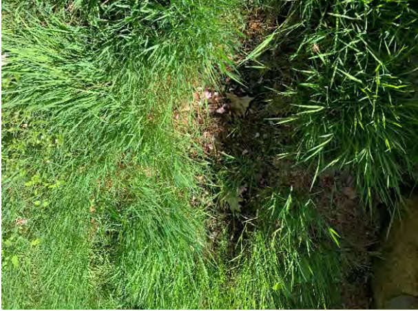
4 Brickyard Circle – 3 (Drainage Course)
